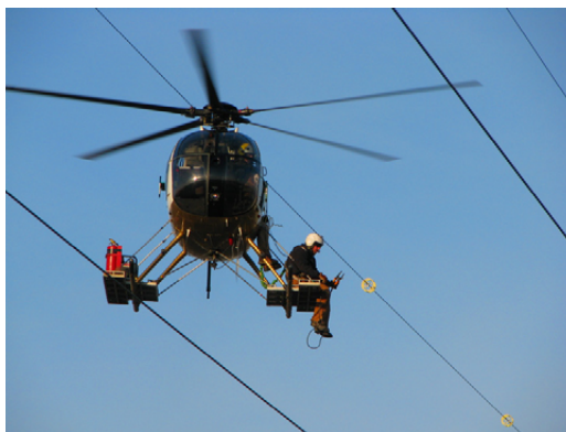
Fig. 2.1: Helicopter Power Line Inspection (Ref. 8)
